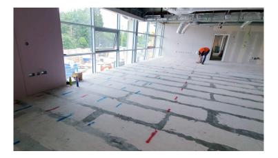
latex layer. The team had to carry out a thorough clean of the concrete surface to allow optimal adhesion of the tape.
