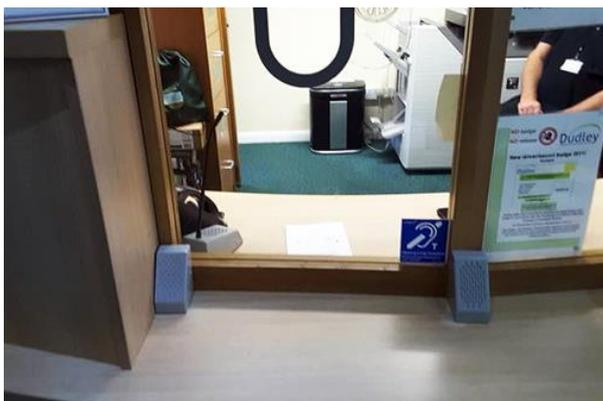
A Contacta engineer visited the school, using specialist equipment to ensure the new Dual Surface Mounted System (STS-K002-(G/B)-01) is fitted neatly onto a countertop. The hearing loop inside of the main reception was replaced with new cables and connections.
