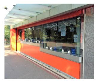
Visitors have protection from the weather when paying for admittance at the ticket office. But the canopy causes a high fluctuation in noise levels as well as echo reverberation.
